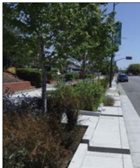
SFEP has led Low Impact Development efforts on both sides of San Francisco Bay. In San Francisco’s Bayview district, SFEP helped the 1700 block of Newcomb Avenue become the city’s first true green street. The makeover, completed in 2011, included stormwater-filtering planters and drought-tolerant street trees. Another LID project installed 19 vegetated stormwater-treatment cells in downtown El Cerrito in 2010, the cells, planted with drought-tolerant native species, slow down runoff and remove pollutants before stormwater reaches Baxter and Cerrito Creeks. Photo by Josh Bradt.
