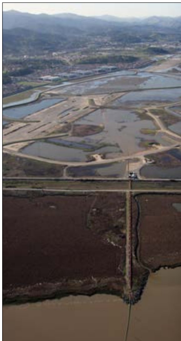
More than five million cubic yards of sediment dredged from the Oakland Harbor deepening project and maintenance projects around the Bay gave this 960 acre wetland restoration site at the former Hamilton Army Airfield a much needed lift. The material had to be pumped five miles across Bay shallows in a pipe especially created for this purpose (bottom center of photo). After years of clean up, dirt moving, and implementation of a complex habitat design, Hamilton's builders hope to open the site to tidal action in 2014. The dredged material helped bring the site up to elevations where marsh plants could take root. Without the long term commitment of the Corps, the Coastal Conservancy, the Port of Oakland, the LTMS program and other partners, Hamilton would not be the showcase of large scale landscape restoration through public-private collaboration that it is today. Photo courtesy USACE.
