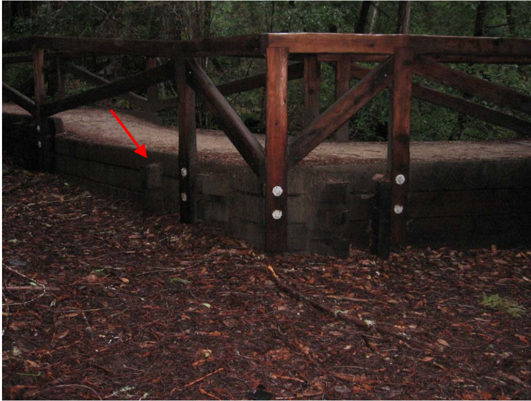
Temporary bench mark
