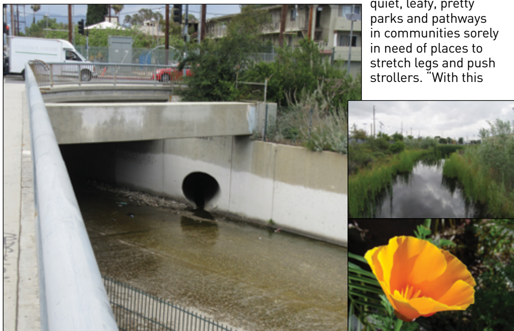
A stormdrain and flood control channel in Tuyunga Wash, an early stormwater recapture project; South Los Angeles Wetland Park. Photos: Tira Okamoto & Wikimedia (poppy)
