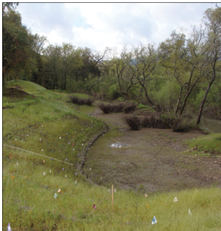
Restored floodplain, willow baffles, and preserved riparian structure on Honig riverfront designed by ESA. Photo: Jorgen Blomberg
