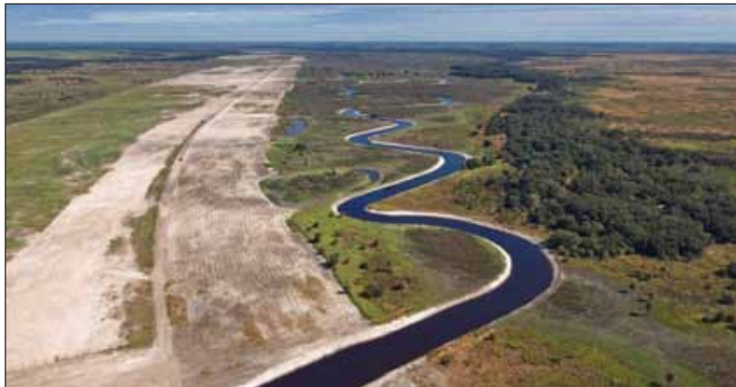
The C-38 canal, backfilled to reclaim the floodplain and meandering oxbows of the original Kissimmee River. Courtesy South Florida Water Management District.
