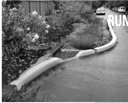
A curb cut directs stormwater into a curb extension "wetland." Courtesy of City of Portland.
