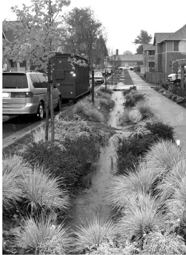
At the High Point redevelopment project, a vegetated swale in the public right-of-way slows and treats runoff. Photo courtesy of Peg Staeheli.
