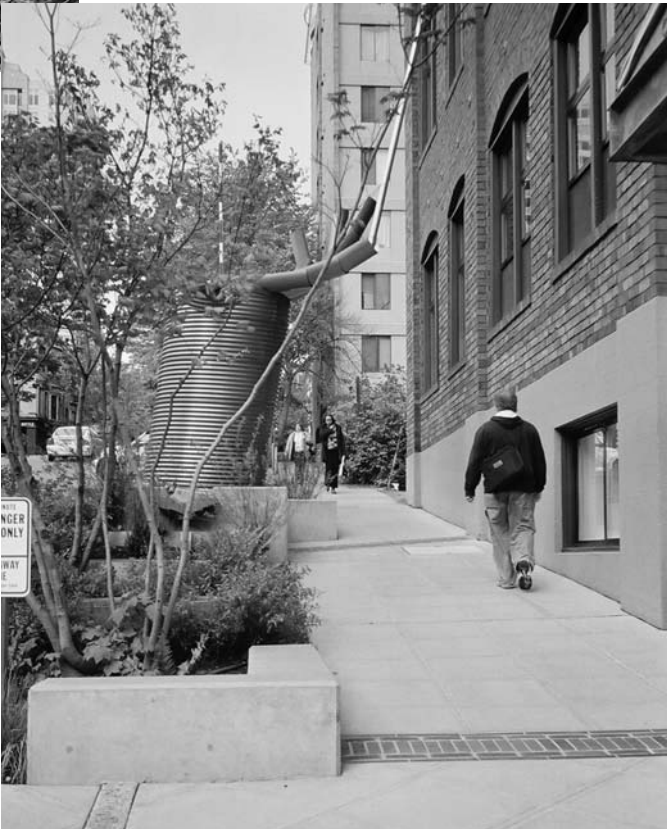
Downtown, a giant cistern captures stormwater and releases it slowly into a series of vegetated pools. Photo by Lisa Owens Viani.
