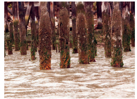
Over 33,000 derelict pilings can be found throughout the Bay. While they offer surfaces for creatures like mussels and oysters to attach to, the creosote they were treated with can be toxic.
