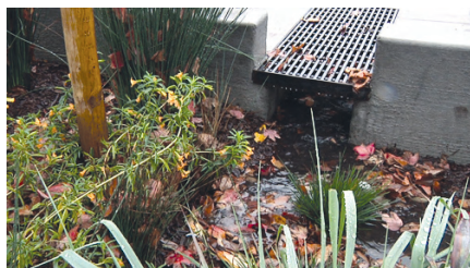
Curb cuts send street runoff into stormwater planters, El Cerrito.
