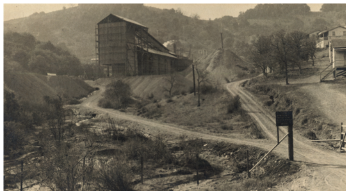
The Senador Mine reduction works, circa 1900, where miners separated quicksilver, aka mercury, from slag. Mercury comes from the red ore called cinnabar. Mexicans began mining the New Almaden district just before the Gold Rush. In its heyday, the district contained hundreds of miles of mining tunnels, several small towns and 1,800 homes for miners—all working to produce and export flasks of liquid mercury. The creek in the photo was one of more than 80 miles of streams that drained the mining area into the Guadalupe River watershed and San Francisco Bay. Photo courtesy History San Jose.
