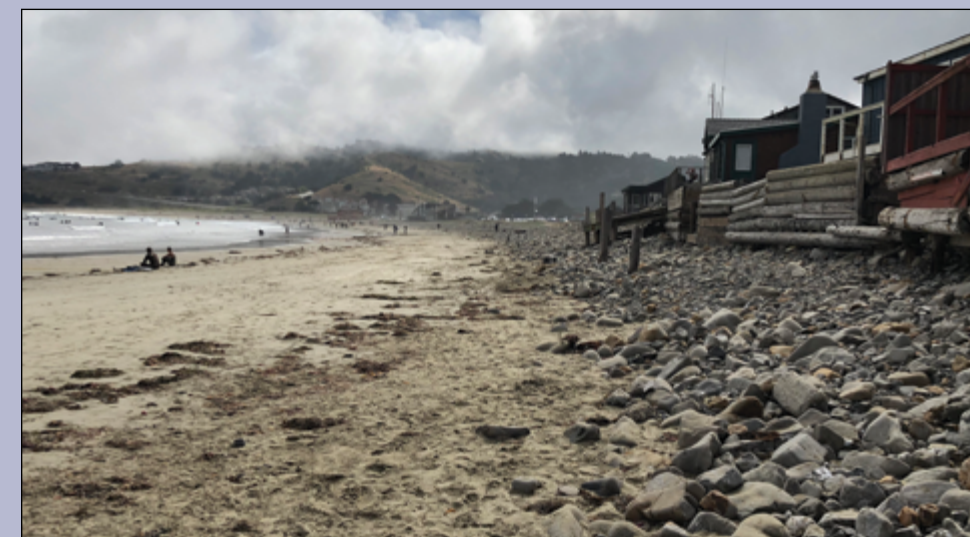
A rock berm guards waterfront homes from high tides and waves at Pacifica State Beach, better known as Linda Mar. The small community, and the nearby shopping center, are a nexus point of community politics and climate engineering as sea-level rises. Photos: Alastair Bland
