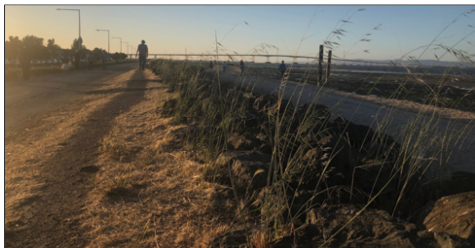
In 2018 Foster City voters approved a $90 million general obligation bond to fund raising the city's levee by five feet. Construction is expected to begin in fall 2020. Photo: Adele Thronson
